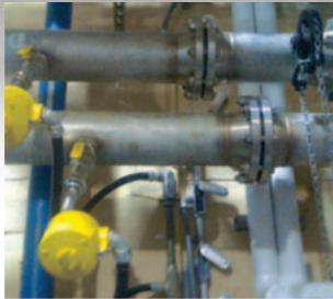
Vortab VMR with flow element installed in optional tap
