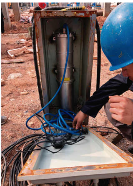
Power Plant, China
