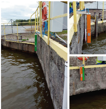
Water Treatment Plant, Estonia
