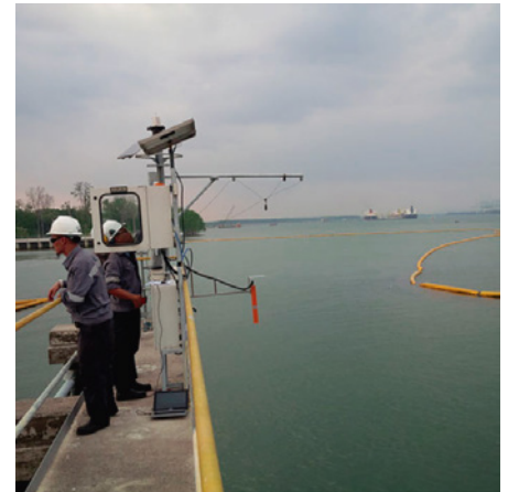
Power Plant, Malaysia
