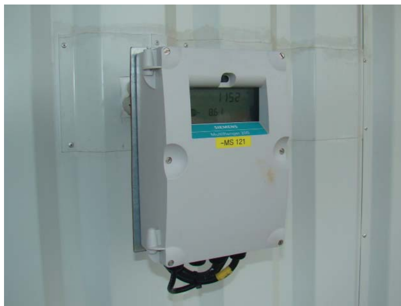
The MultiRanger 200 provides continuous and precise level monitoring for Sattler AG's gasholders.
